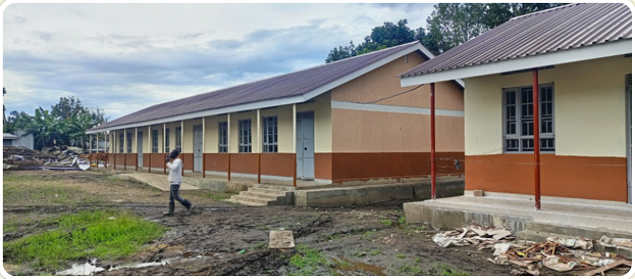
The completed classroom blocks at Bukuuku Community Seed School
