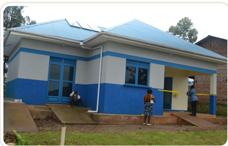
A water house at Mugusu sub county constructed under LEGS programme
