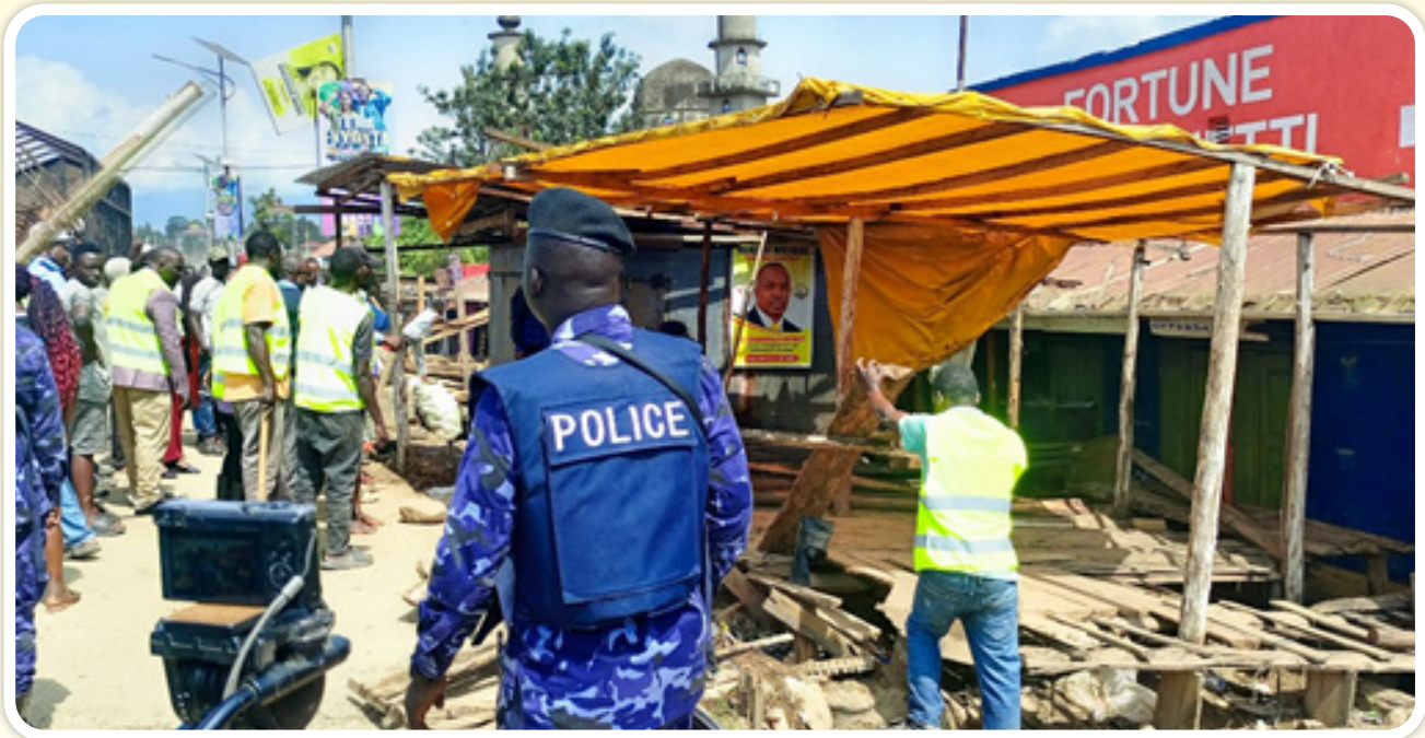
Demolishing the illegal structure in Kisenyi area
