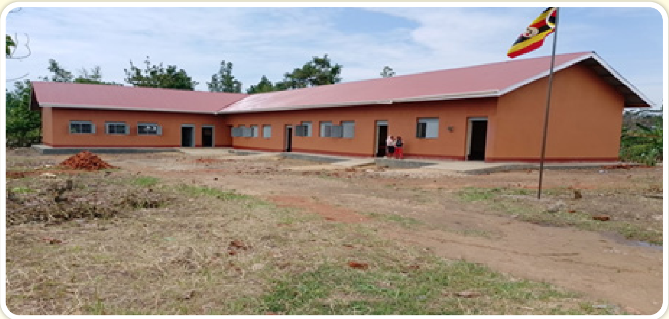
A new 4-classroom block with an office and staffroom at Kinyante Primary School
