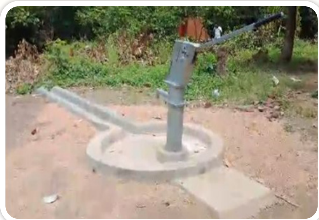
A fully functional water borehole constructed at Kinyante Primary School
