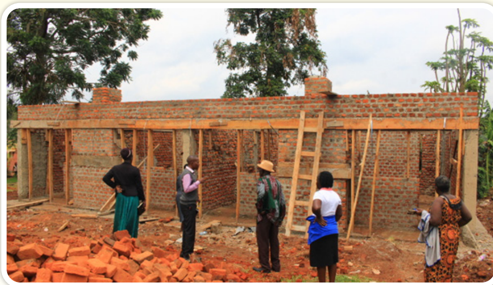
Ongoing construction of staff quarters at Kisojo HC III
