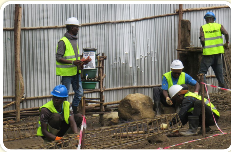
Ongoing construction of the Visitor Information Centre.
